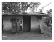
during rainy season because water enters in to the house and there are leaks in the roof. There are no doors and windows. It is not at all safe to sleep inside the house. It can be fallen at any time. The floor of the house is covered with mud. The walls and floor of the house are severely cracked. She fetches water from a public well about 1 km away from her house for all household purposes. They have 0.04 acres of land as her own. Their dream is to have a small and safe house as their own.
